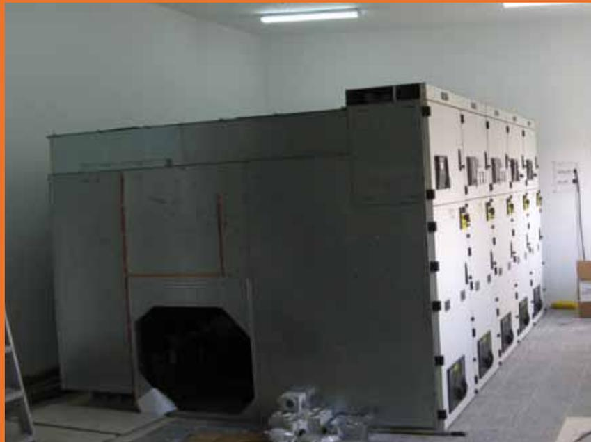
Due to the oldness of this station and its small size , 33 KV switchgear was replaced by new one in addition to extending the building and its capacity to 30 MVA .
